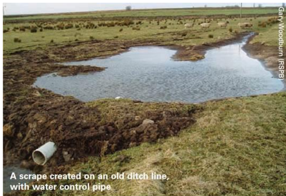
Figure 8: Scrape Connected to Ditch Line (RSPB Guidance) 18
